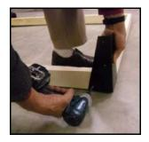
3. Fasten the front lift bracket raising the front of the coop and propping it high enough so as to drive the fasteners into the bottom of the front rail.
