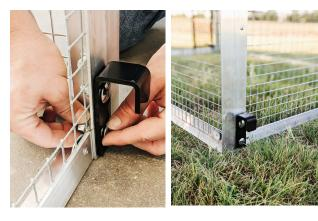
5. Fasten front hooks using four 3/8" X 1" carriage bolts. Carefully straighten the hooks before tightening bolts with 9/16" wrench or socket.
