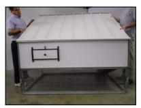
10.) Position the roof section on the angle frame, sliding it toward the back until the wooden frame rests inside and against the angle frame. The side with the ceiling hook should be toward the front. This allows approximately 3 1/2" of overhang on the front and back sides. Center the back of the roof from end to end leaving it nearly even on each side.
