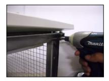
**12.)** Square up the front of the roof on each side and fasten the two front corners with 2" wood screws.
