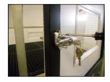
**8.)** Install the T-handle latch on the outside of the right door with the screws provided.
