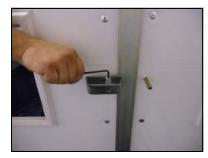
**9.)** Turn the T-handle to the vertical position and install the inside catch horizontally so that the short side of the D-handle overlaps the center doorstop. Tighten it with a 1/8" allen wrench. Follow the same procedure on the other door.
