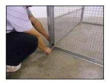
**5.)** Using a 9/16" socket and wrench, firmly tighten the eight bolts holding the frame in place, carefully aligning the corners of the Egg Cart'n.
