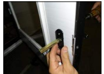
8.) Install the T-handle latch on the front door using the backer plate on the inside.
