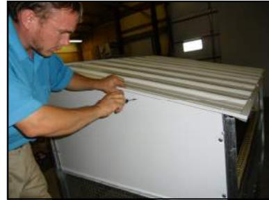
7.) Using 1 1/2" screws, fasten the roof through the holes at the top of the end pieces. Tighten the eight 3/8" bolts that hold the frame in place with wrenches.
