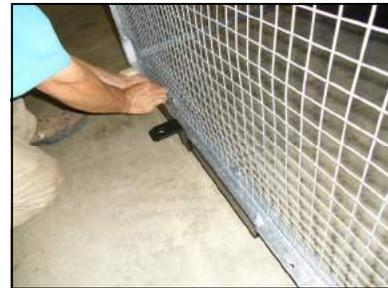
15.) Install the front lift bracket with two 3/8" x 1" hex bolts.
