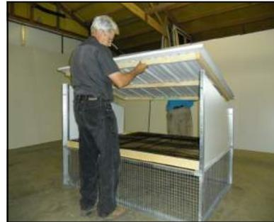
6.) Position the roof on the unit, paying attention that the angle cuts on the roof frame match the vertical angle pieces of the side and end pieces.
