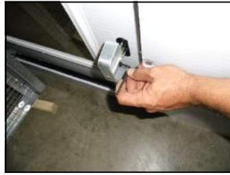
9.) Install and adjust the D-handle so that the door is snug when closed.
