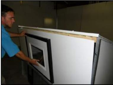
10.) Position the front panel and fasten it with 1 1/2" screws.
